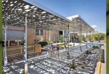
Image of Perforated Panels
