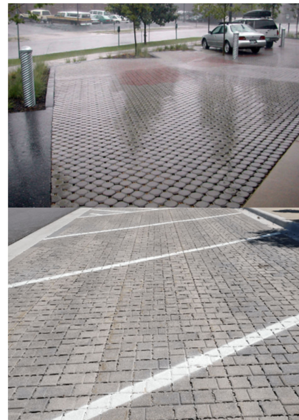
Fig. 9 Example of Permeable paving surface concepts
