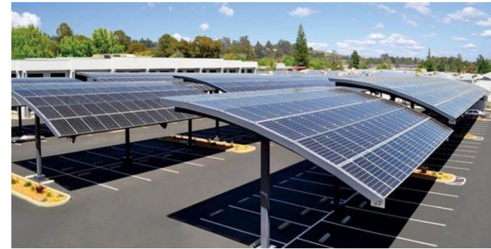
Fig. 7 Example of Solar parking canopy structure
