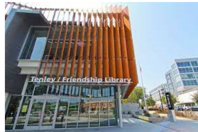
Vertical louver sun control
