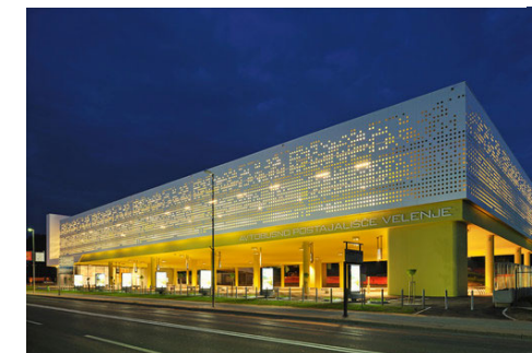
Fig. 21 Example of perforated screen used for parking garage
